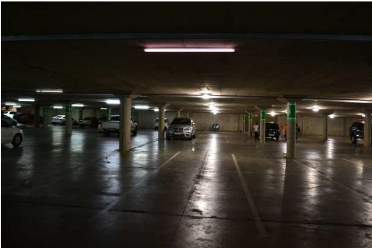
Above is a pilot project in the undercover parking area of a local shopping mall where we installed 20 of our 40 Watt induction bulkheads. These replaced on a one for one basis the existing 2 X 35 Watt open channel T5 fixtures. The bulkheads are on the right and the T5's are on the left.
